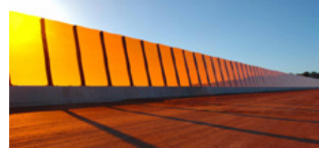
RESILIENCE AND SUSTAINABILITY: Noise wall, EastLink Freeway, Melbourne.
