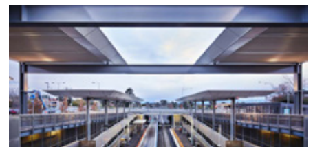
SAFETY: Mitcham railway station, Melbourne.
