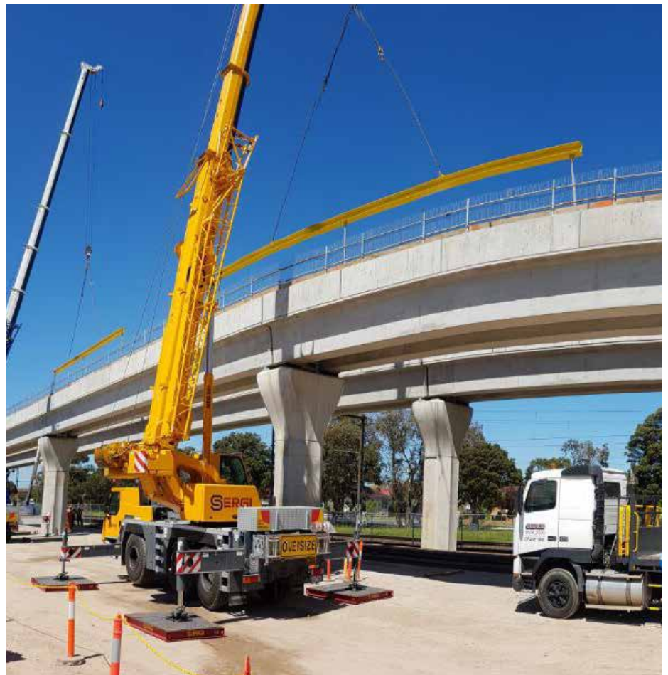
Rail being placed on elevated structure near Ross Reserve.
