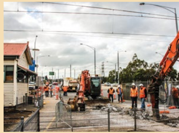
Early works to construct the Burke Road bridge deck
