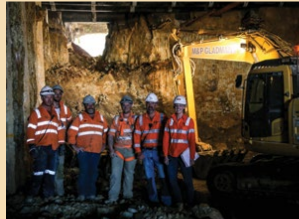
Break-through excavations underneath Burke Road
