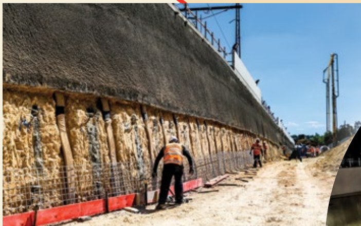
Reinforcing the rail cutting
