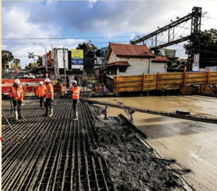
Pouring the concrete bridge deck
