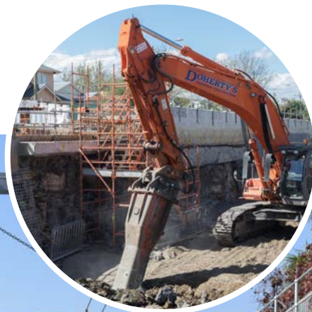
Rock breaking and trench excavation (left), and the completed rail trench and road bridge (below).
