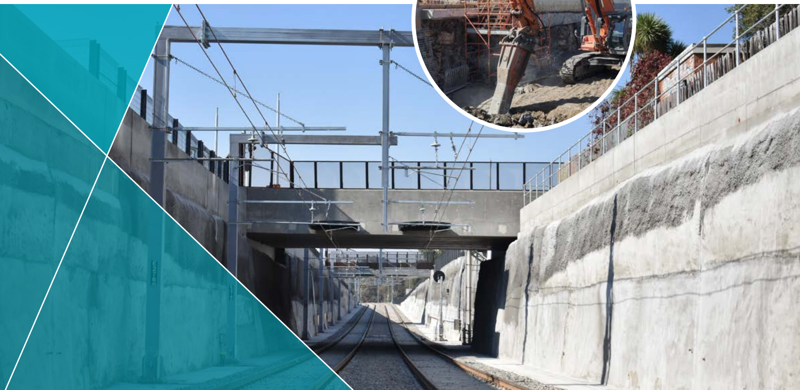
Rock breaking and trench excavation (left), and the completed rail trench and road bridge (below).
