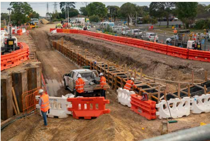
Sneak peek as construction begins on the new underpass
